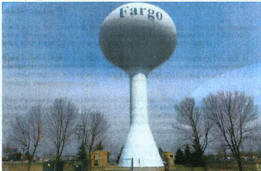
Water Tower Number 7 (1 million gallon capacity)
