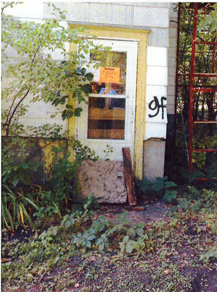
703 10 Ave. N., Fargo, ND 58102—Dangerous Building Notice and Graffiti 8/16/18
