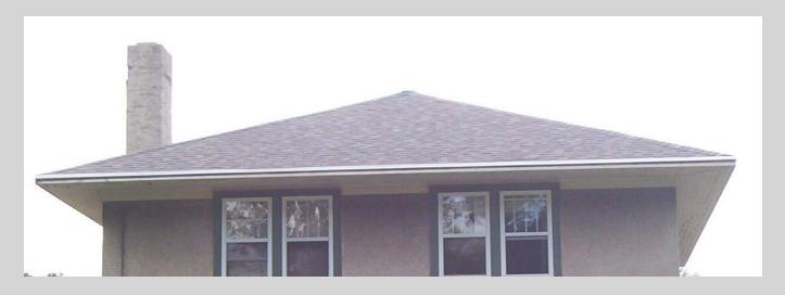
This is an example of a **hipped roof**. The minimum pitch for a hipped roof is 4:12. A pitch of 4:12 means that for every 4 feet of vertical measurement to the peak, there is a horizontal measurement of 12 feet.
