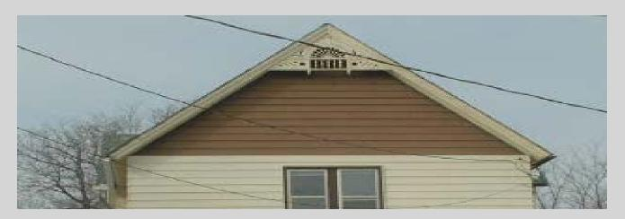
This is an example of a **gable roof**. The minimum pitch for a gable roof is 6:12. A pitch of 6:12 means that for every 6 feet of vertical measurement to the peak, there is a horizontal measurement of 12 feet.
