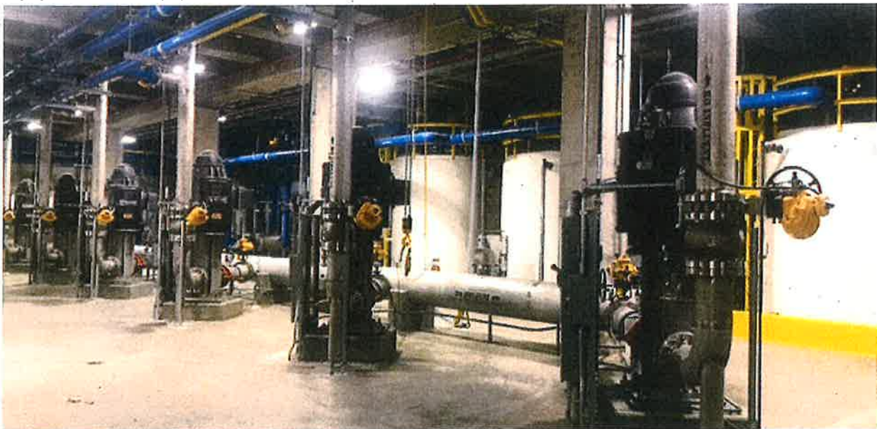
View of Reverse Osmosis (RO) Pump room on the lower level of the MWTP. RO pumps and RO cleaning systems are shown in the picture. Photo from January 2019.
