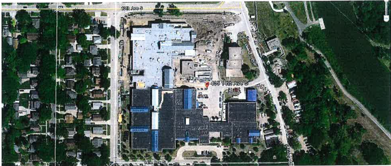
Google Earth view of the existing WTP and the MWTP prior to membrane roof replacement.
