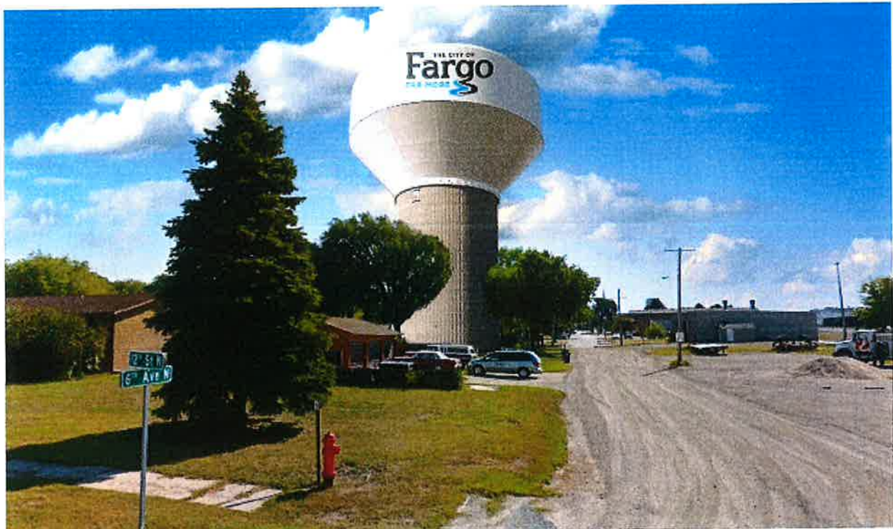
New Downtown Water Tower listed for funding in 20-year CIP with SRF loan program.
