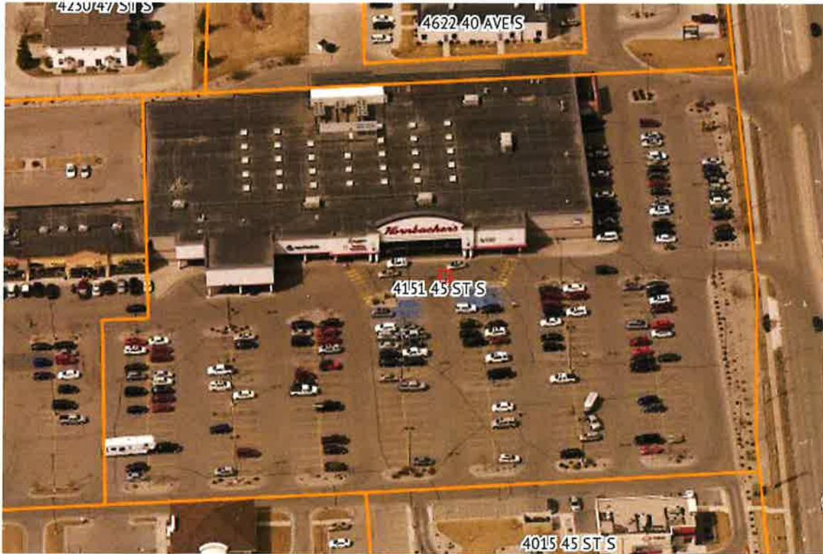
Subject Property (Looking West)
