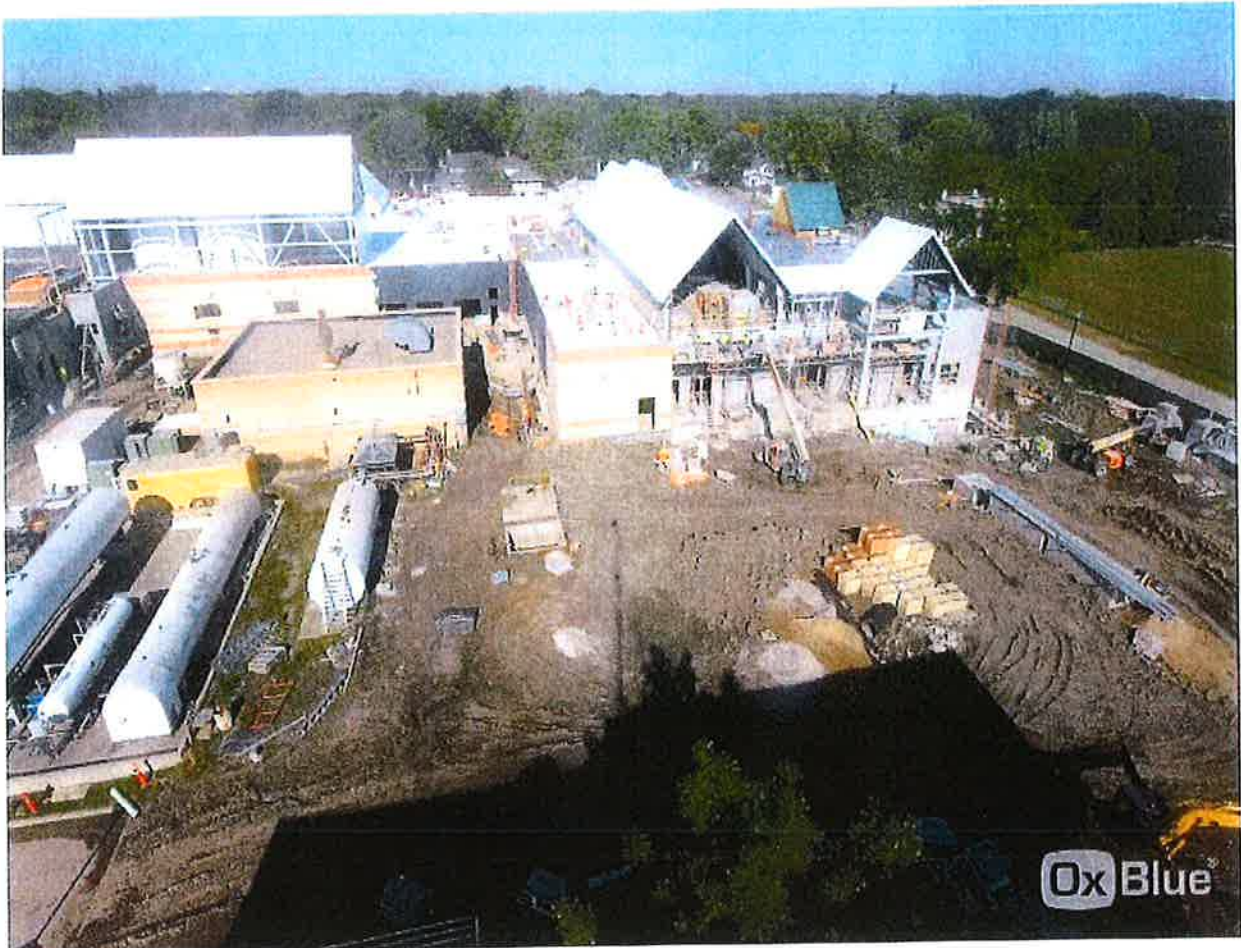
Overview of Fargo MWTP construction. Picture is from August 7, 2017.
