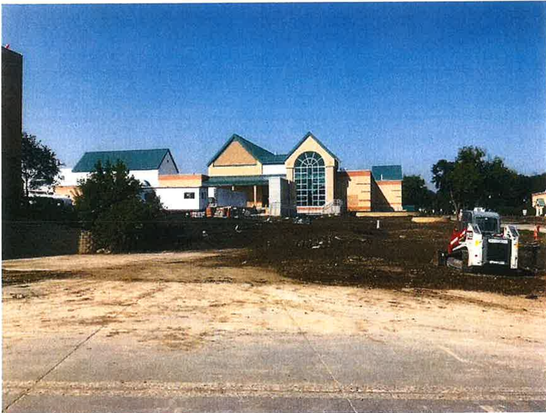
View of MWTP and Residuals Facility from 4 th Street South. The storm water retention system, Red River raw water pipe, and electrical infrastructure are underground in this area. Change orders related to modifications in this area are included in the recommended contract changes. Photo from August 2018.
