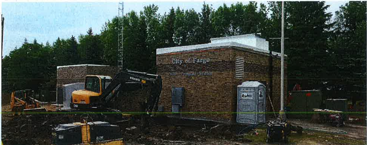
Sheyenne River Pump Station with new electrical building under construction (Summer 2018).
