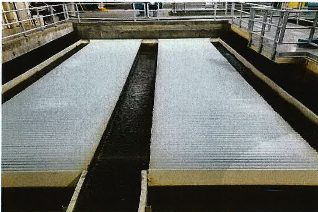
Plate Settlers in the Pretreatment Process of the Lime Softening Water Treatment Plant.
