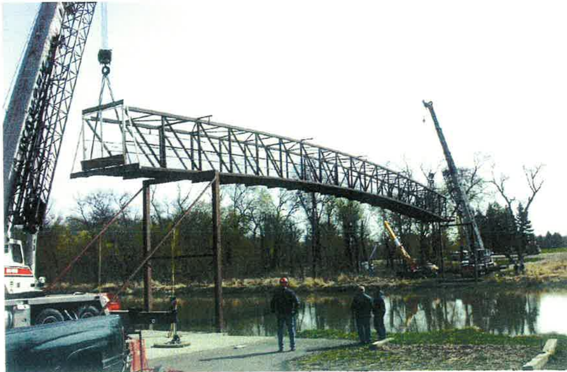
Figure 3: Bridge Removal
