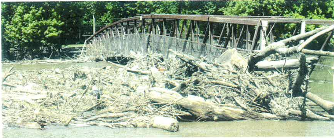
Figure 2: Seasonal Flood Damage
