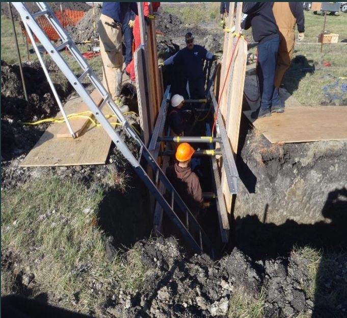
Trench Rescue Training
