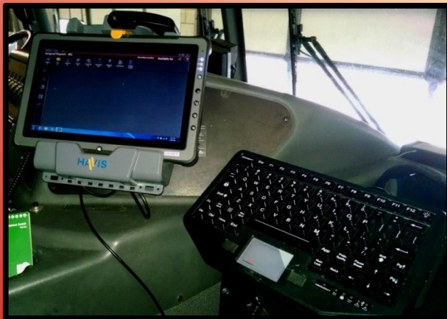
Getac Computers have been mounted in each unit for receiving calls from dispatch and getting information on scene.
