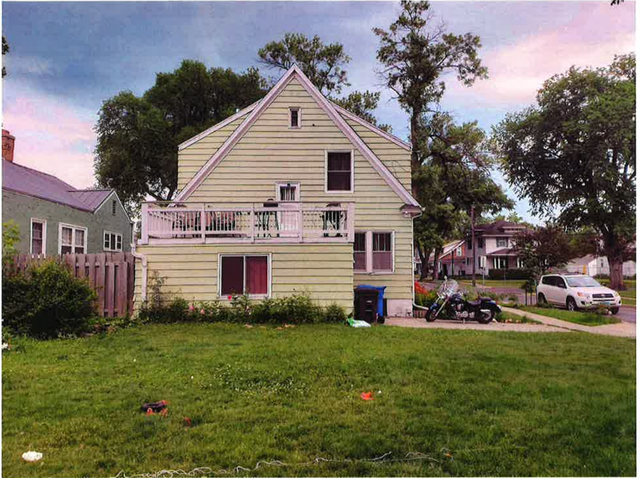
West side of House
