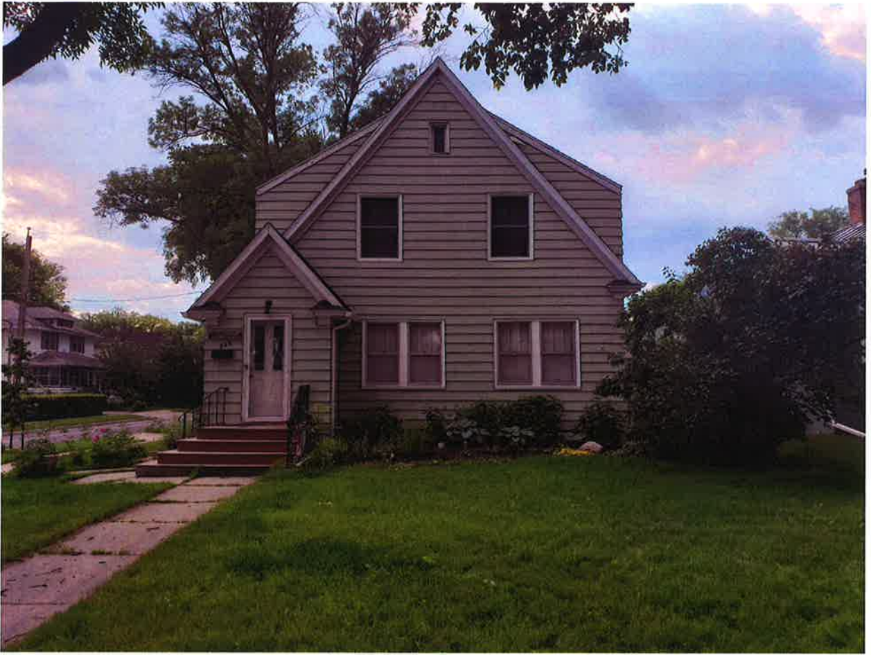
West side of house
