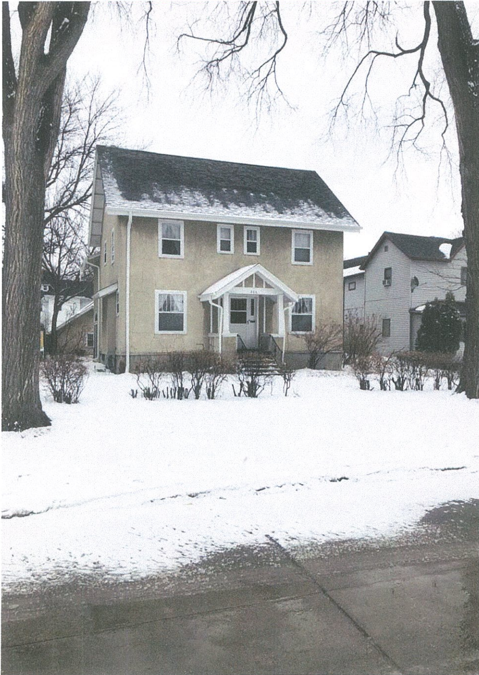
West elevation of house - Front
