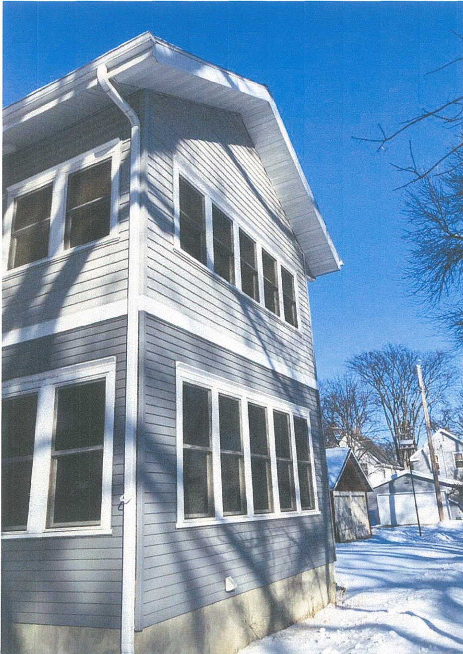
South Elevation (Street Side) of House
